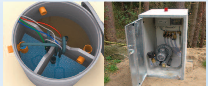
Control Cabinet ZINK SBR Plant 50 residents
