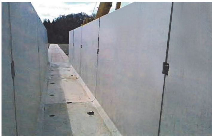
Mobile silage wagon panels, which are each structurally connected by three BT turnbuckles and are immediately ready for use
